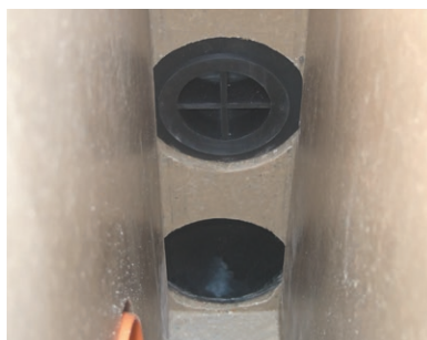
View of foul air trap before installation
